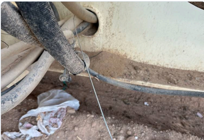
A fish tape makes pulling wire through tight spots easy.
